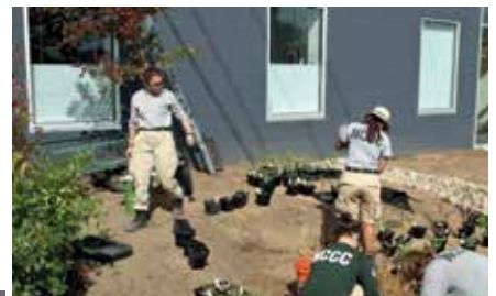
RAIN GARDENS Rain Garden Installation at Watermark Art Center
